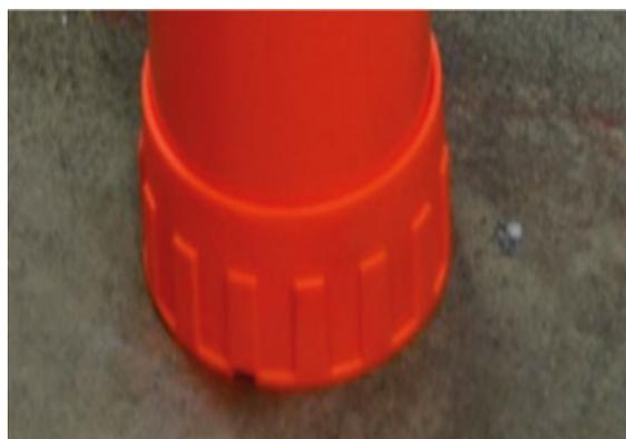
Once the epoxy has fully cured you can remove the City Post from the anchor cup. If the steps are followed correctly and in the shown sequence, you should have an installation that looks very similar to this.
