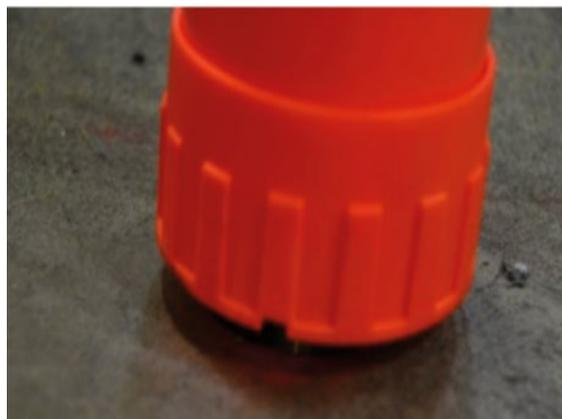
Once the final depth is reached no adhesive should be visible around the base. Allowing the anchor and epoxy to set, refer to your manufacturer's direction for cure times.
